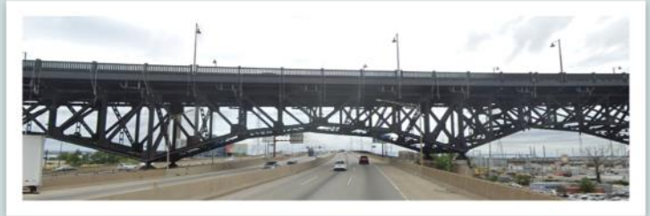
Figure 2 - Pulaski Skyway over the NJ Turnpike Easterly Alignment
