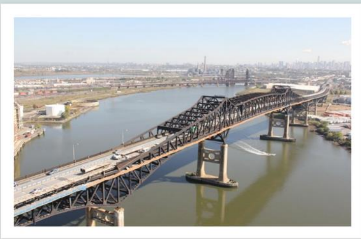
Figure 1 - Pulaski Skyway (Passaic River Crossing)
