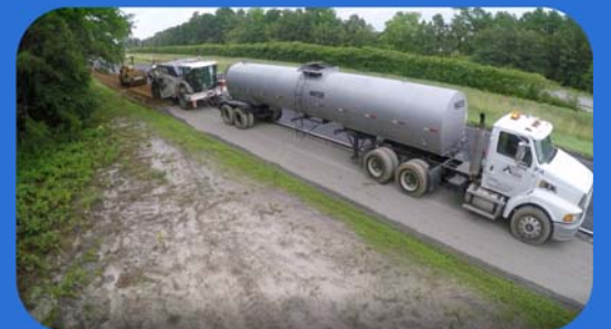
FDR Equipment Train on Rt. 55 SB
