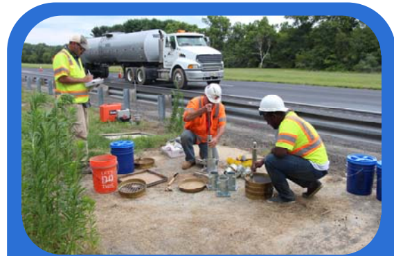
AID Material Testing Team Performing QA Testing for FDR on Rt. 55 SB (left to right: Hasan Neamah, Inspector, logging sample information; Dan Nero, Senior Technician, molding FDR Samples for compressive strength; Ahmed Mohamed, Engineer, preparing sieves for gradation control)
