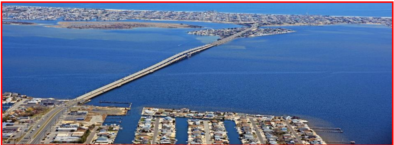
Route 37 Mathis Bridge over Barnegat Bay connecting the New Jersey mainland with beach communities such as Sea Isle City
