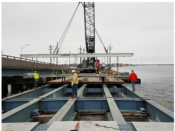
Exodermic deck reconstruction
