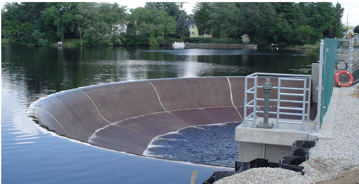
Malaga Lake Dam – 2004 Distinguished Award for Engineering Excellence, ACEC/NJ
