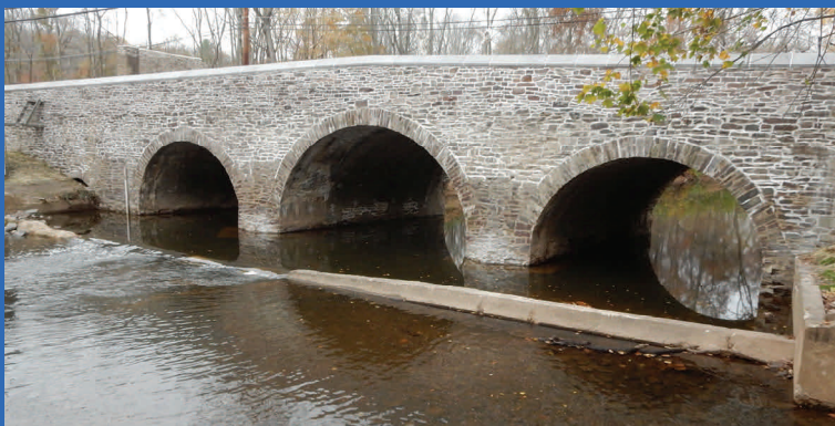
Completed Stone Arch Bridge
