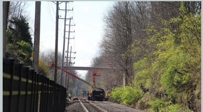
Low clearance power lines supplied essential power to a medical center procuring COVID-19 test kits. Beam installation was coordinated when another energy source was brought online to power the facility
