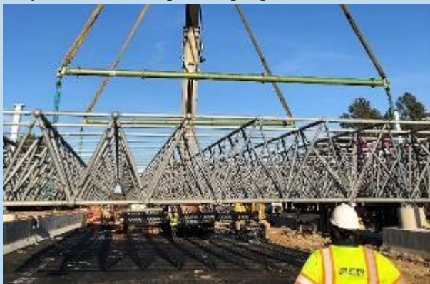
New Canopy for the New Gretna Toll Plaza
