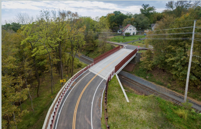
New bridge design has two lanes with shoulders in each direction. New crashworthy bridge railings, guiderails, and aesthetic fencing elements that respect the original site’s settings
