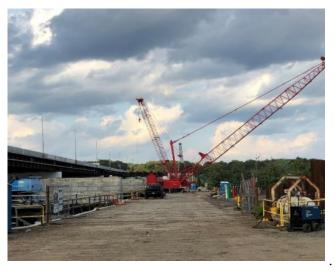
Mr. Skeels explained that the Contractor, Trumbull Corporation was able to make an important adjustment to the of the trestle causeways design, raising the grade to match the adjacent River Road, and allowing better access to pier work. This approach required the Contractor to receive expedited approval from regulators. The tour allowed participants to see pier construction in various stages of completion.
